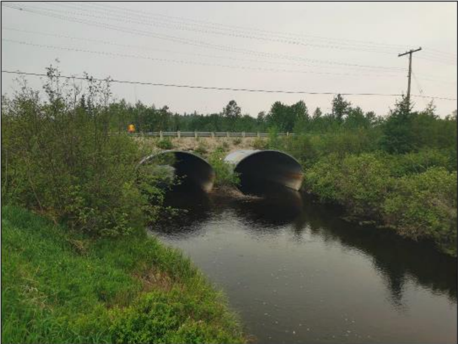
Picture 4 – East Elevation
