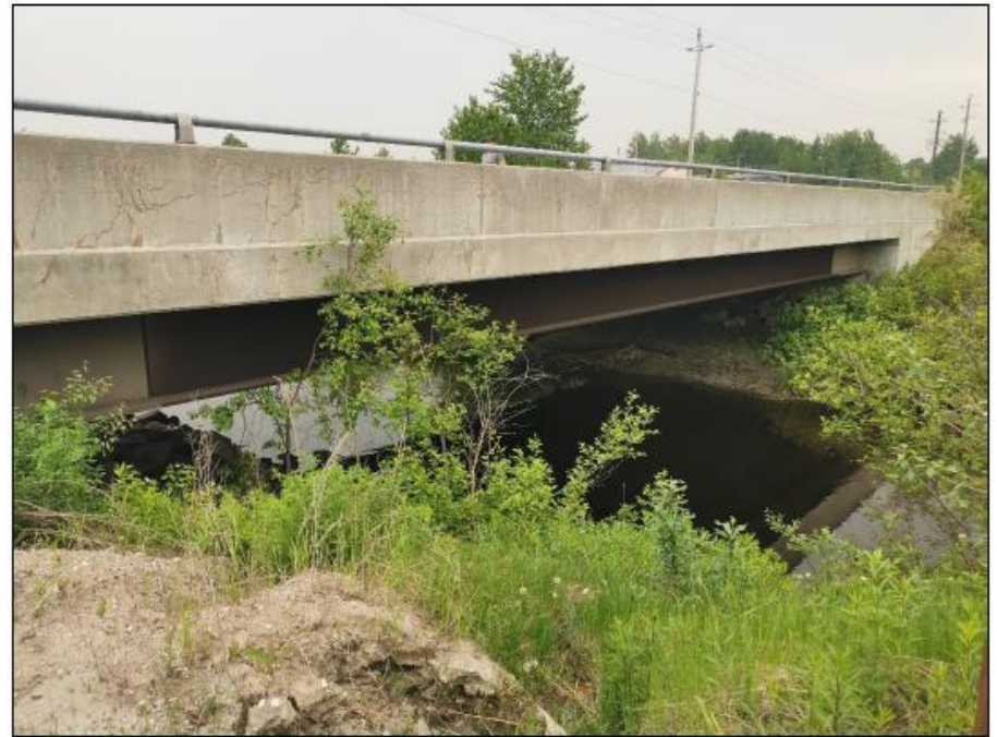
Picture 4 – North Elevation
