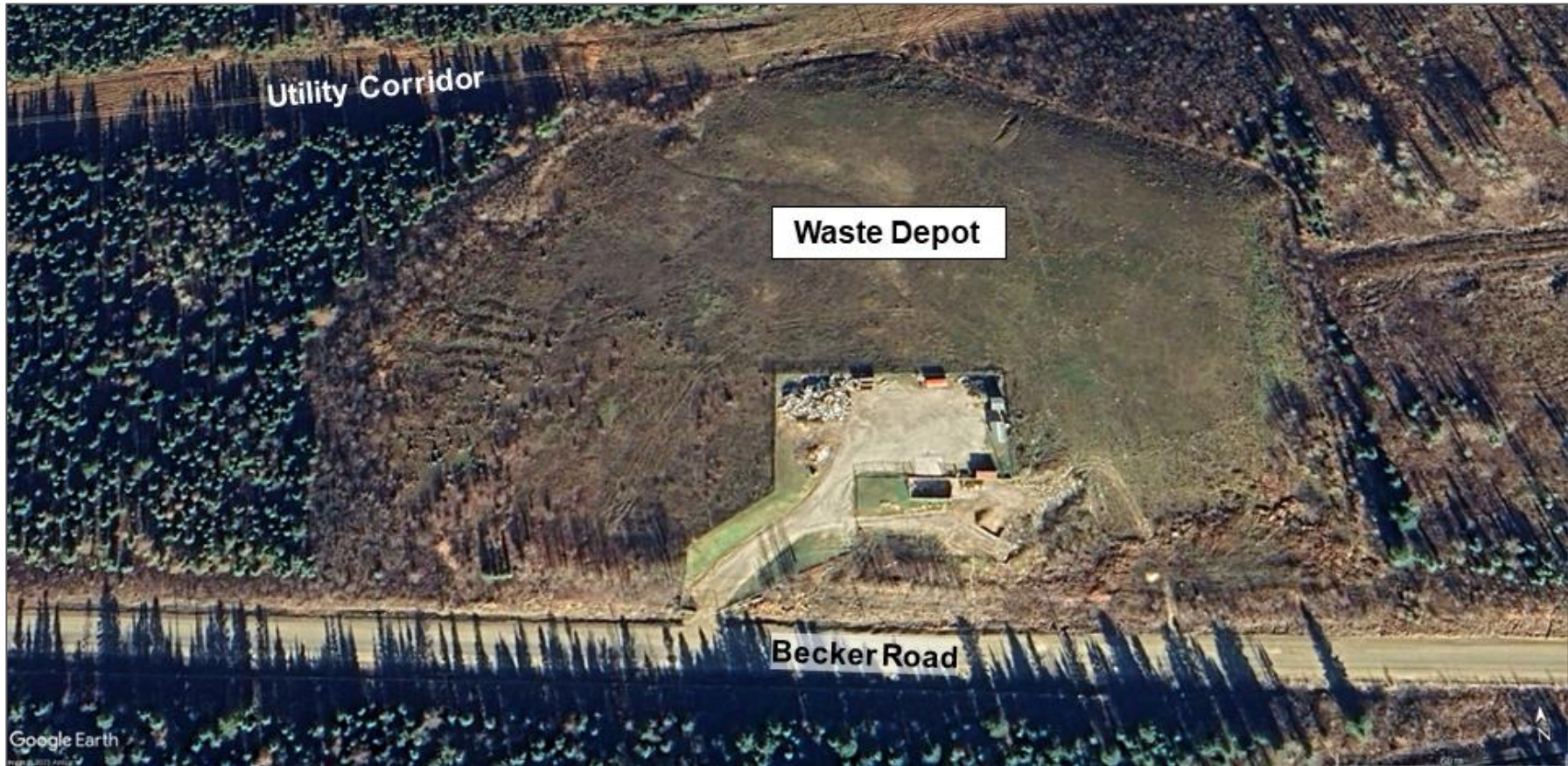
Figure 8: Hornepayne Waste Depot
